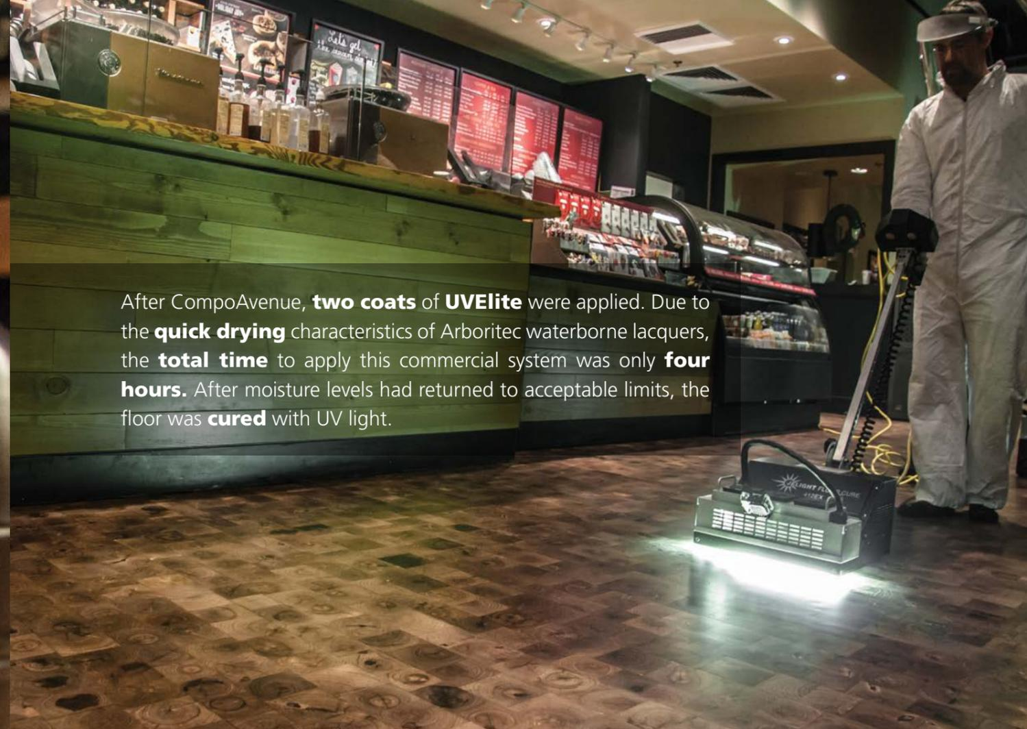
After CompoAvenue, **two coats** of **UVElite** were applied. Due to the **quick drying** characteristics of Arboritec waterborne lacquers, the **total time** to apply this commercial system was only **four hours**. After moisture levels had returned to acceptable limits, the floor was **cured** with UV light.
